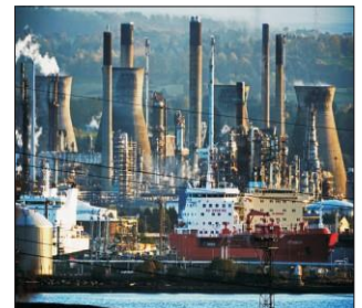
Refinery Petrochemical Plant
